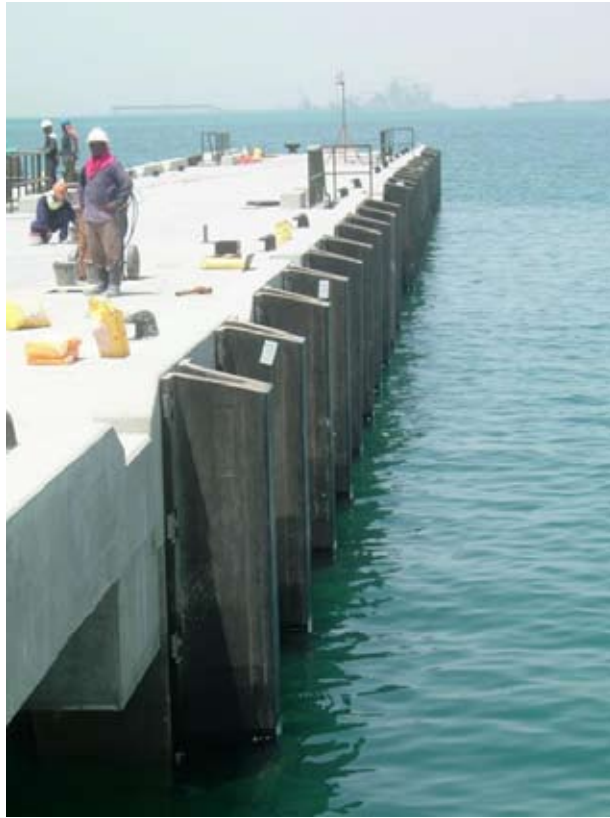
FIGURE 3 Zeron 100 fasteners attaching rubber fenders on a Middle East dock.
