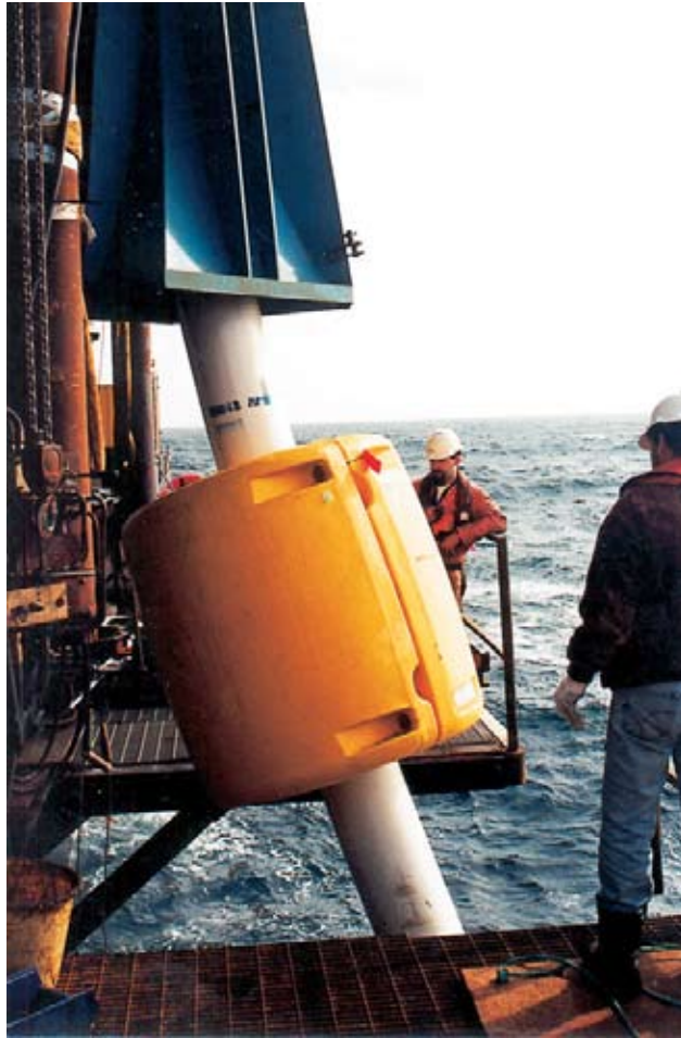
FIGURE 2 Deployment of riser with buoyancy modules.
