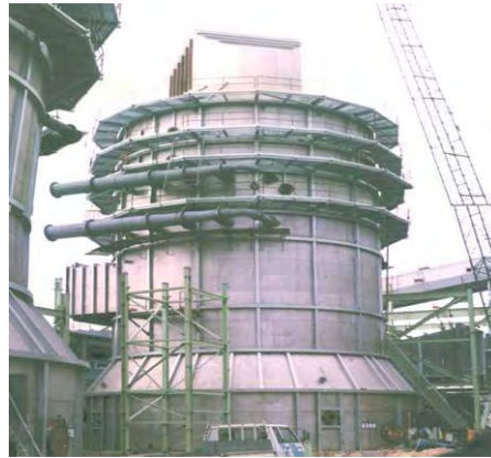
Figure 11: Absorber tower at KEPCO Hadong power station.
