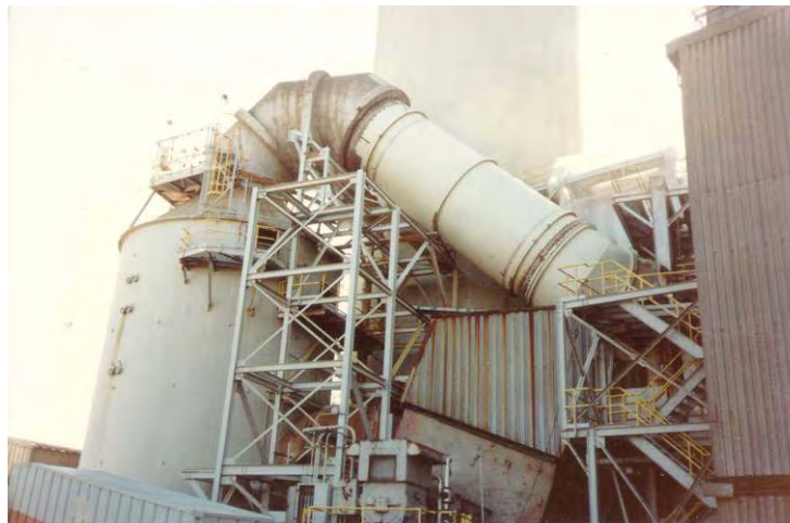
Figure 10: LG&E Cane Run #6 Absorber Tower and Downcomer
