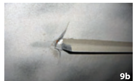
Fig. 9a. & 9b. Example of a calciner unit that suffered cracking of the shell. This was a result of temperature differentials between the shell and internal flights.
