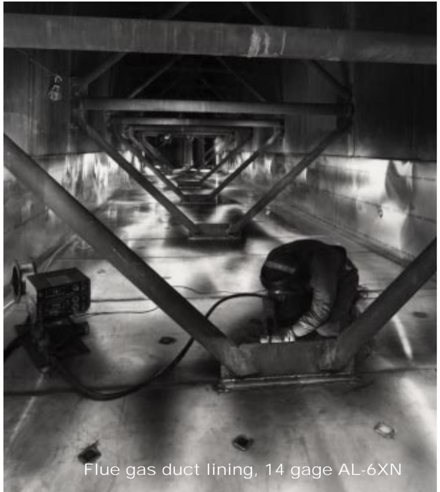
Flue gas duct lining, 14 gage AL-6XN
