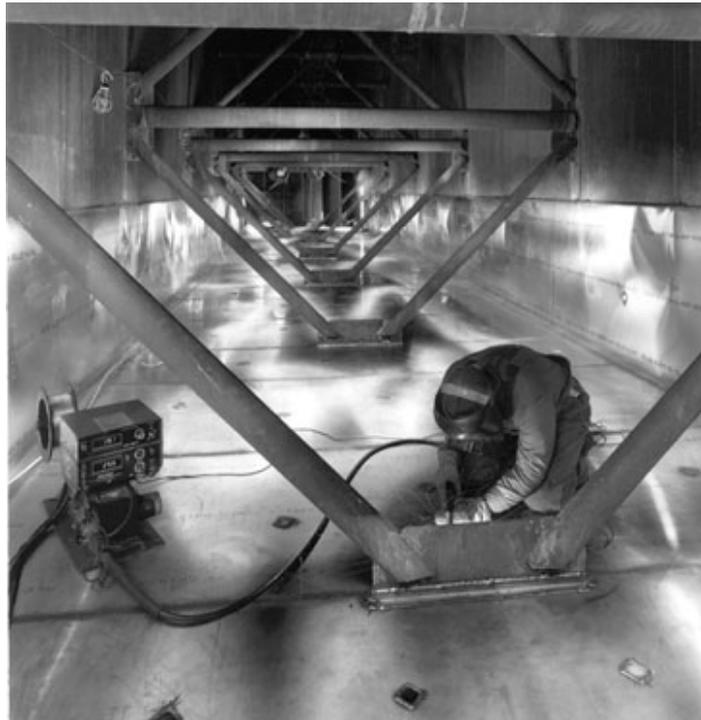
Figure 7 – AL-6XN was used for the wallpapering of a carbon steel duct connecting the electrostatic precipitator to the flue stack. Lower than expected temperatures led to condensation in the bottom of the 12-foot wide duct. Duct was approximately 150 feet long. After 5 years in service, the duct was removed from service with no reported problems. Removal was due to installation of a new wet FGD scrubber system.
