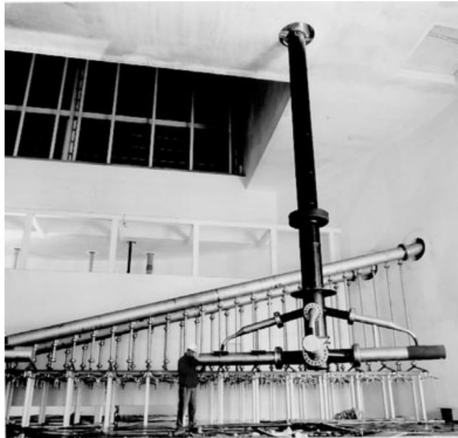
Figure 5 – AL-6XN piping was used for the construction of slurry recirculation piping and rotary sparger unit submerged in limestone scrubber tank. This NIPSCO Bailly Generating Station Units #7 & 8 has used AL-6XN for over 10 years. Environment estimates in the absorber are a pH of 6, 11,000 mg/l chlorides and 130°F.
