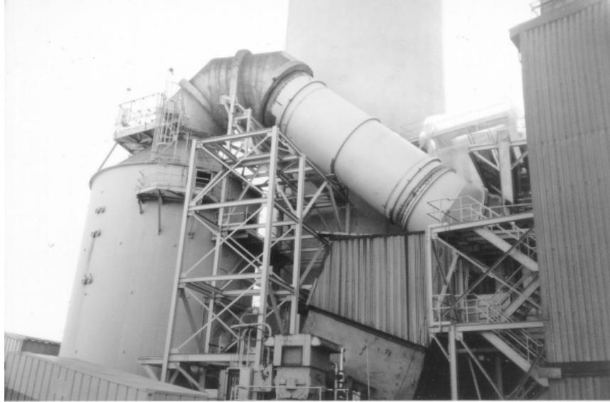
Figure 4 – AL-6XN replaced 317LMN stainless for the lining in two FGD duct systems. 317LMN failed after three years in service. AL-6XN has been in operation after 10 years in service to date. Louisville Gas & Electric was the utility and Cane Run #6 was the unit.
