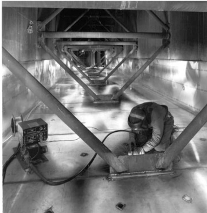
Figure 7 – AL-6XN was used for the wallpapering of a carbon steel duct connecting the electrostatic precipitator to the flue stack. Lower than expected temperatures led to condensation in the bottom of the 12-foot wide duct. Duct was approximately 150 feet long. After 5 years in service, the duct was removed from service with no reported problems. Removal was due to installation of a new wet FGD scrubber system.
