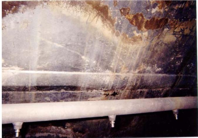
**Figure 5: N08367 Alloy Strips Covering Welds**
