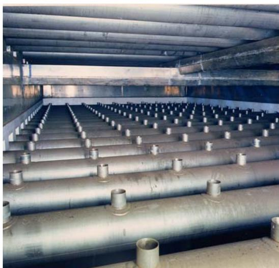
**Figure 3: N08367 Alloy Spray Piping**
