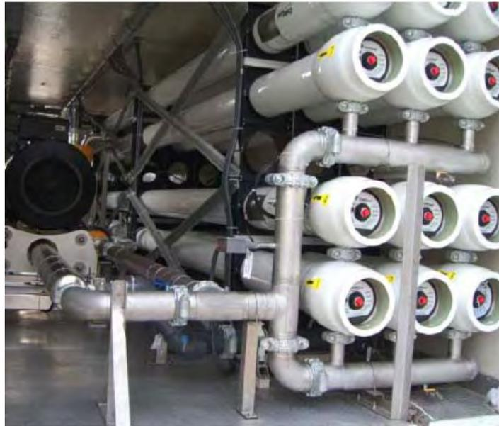
Figure 4 Brine Discharge Piping Using AL-6XN pipe
